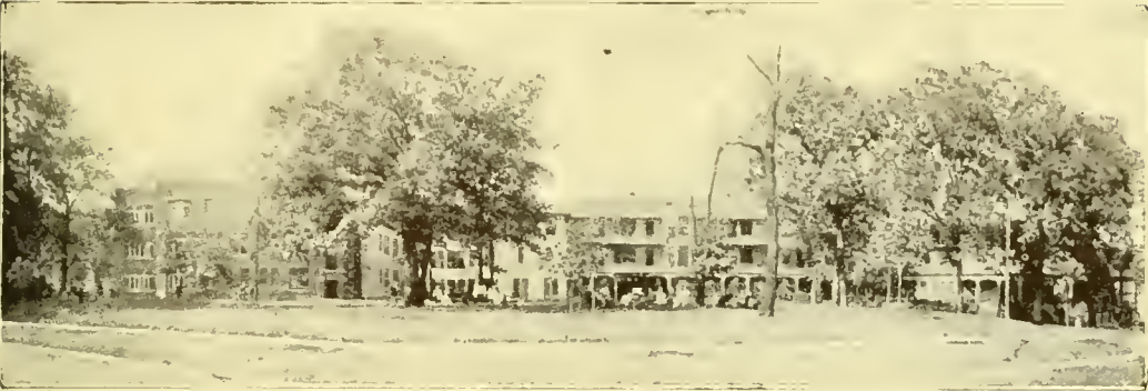
Showing the old building and a part of the new fifty room addition. Capacity 150 patients.
