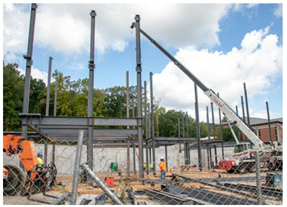
To date, workers have poured nearly 800 cubic yards of concrete and used more than 250 tons of steel, both of which help define the building's shape and future footprint. Steelwork is scheduled to be completed by the end of September. Less noticeable but equally critical progress includes rough plumbing in the slab and soil backfill against the base of selected walls.
