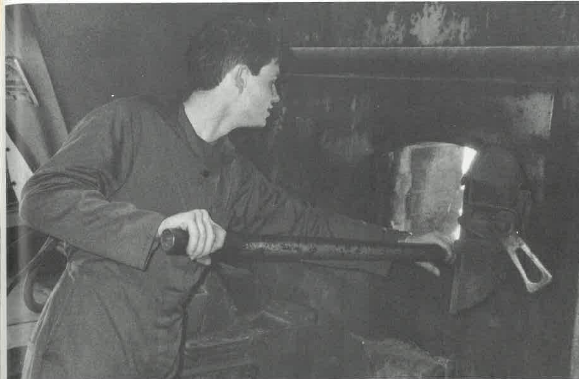
Mike Devlin spreads the coals around as he empties the boiler of old ashes.
