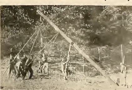
One of the many jobs was that of putting up light poles at the tennis court
