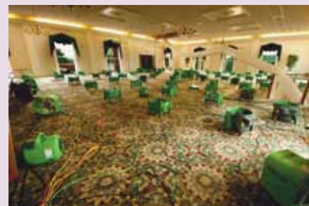
A leaky pipe caused the Dining Hall to be invaded by a small army of green fans over the summer.
