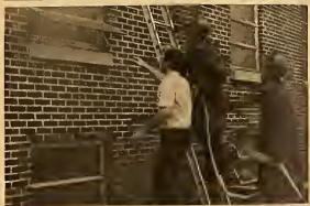
Annoying wisps of smoke emanating from Room 129 of the Women's Residence Hall on Nov. 12, members of the Tri-County Fire Department prepare to halt damage inflicted by electric wall heating unit. Tam Evans, left, gestures at smoke while Lynn Robertson and Buddy Lane hold hose. Despite all efforts, damage did not exceed $300.
