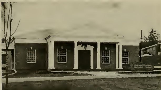
The new Ooltewah-Collegedale Telephone Company building, located on the corner of Camp Road and old Apison Pike.
