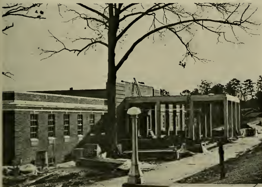
Front view of the new cafeteria which is nearing completion.
