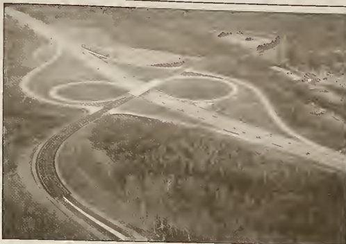
The new, completed Exit 9 off I-75 is waiting to be connected to roads leading into Collegedale and the Enterprise South industrial park. Photo By Brian Brennan
