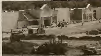
Construction on the Collegedale Wal-Mart continues. The store is expected to open the beginning of 2007.
