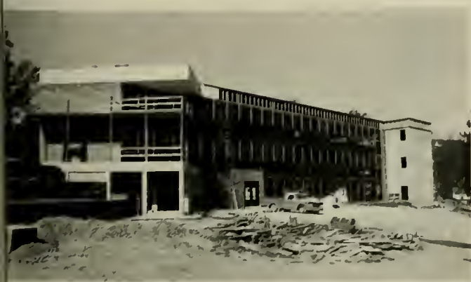
The humanities building under construction.
