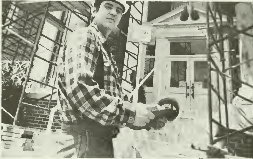
John Leeke pauses during work on the Wright Hall columns.
